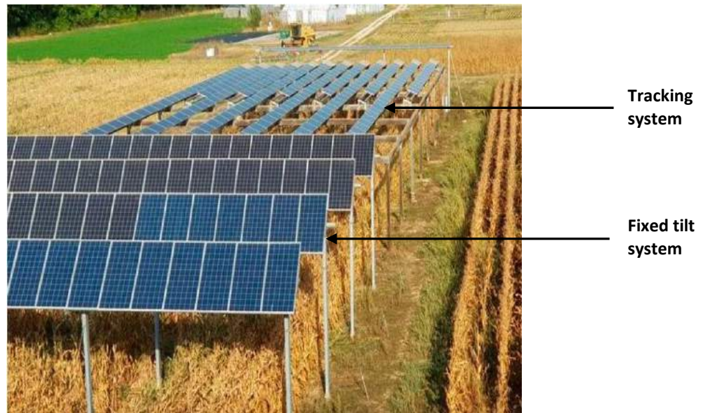
Figure 4. Fixed tilt and tracking systems (Toledo & Scognamiglio, 2021).
