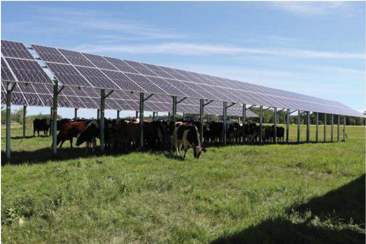
Figure 10. Single pile system at the University of Minnesota West Central Research Outreach Centre (WCROC).
